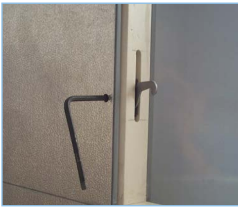
CAM-LOC FASTENING SHOWN WITH WRENCH
